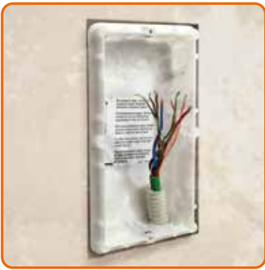
Removal of the existing entrance panel
