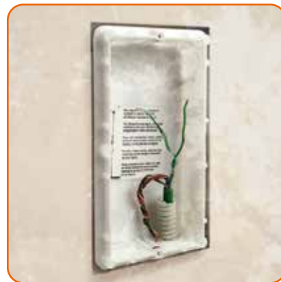
Use of an existing pair of wires to connect the new 2 WIRES entrance panel
