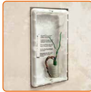
Use of an existing pair of wires to connect the new entrance panel
