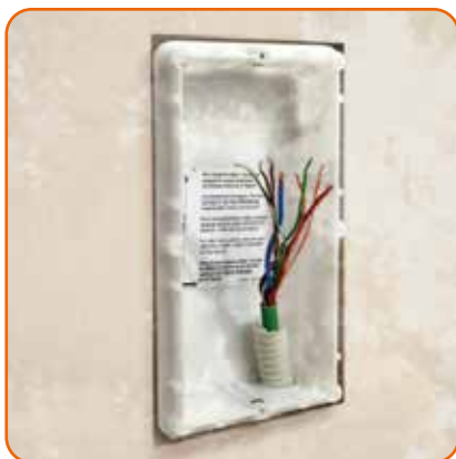
Removal of the existing entrance panel
