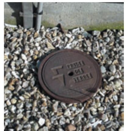
^ Lightning conductor earthing electrode
