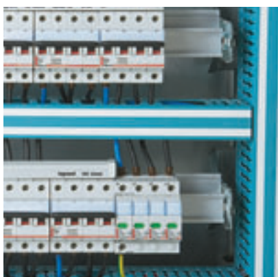
< To reduce the connection length, the associated protection is installed on the row above the voltage surge protector
